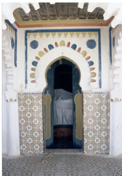
Picture 10 Entrance to Sidi Chaib
