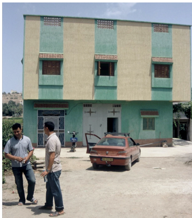
Picture 11 Migrant house in a small Rifian village
