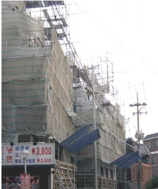
Residential houses were being renovated into office buildings.
