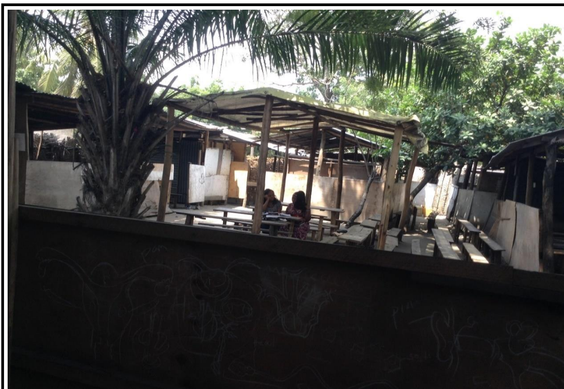
Plate #1 – Description: Premises of one of the private NFSE centres. Six different classrooms (as captured) were formed in a small area on the street’s roadside partitioned by palm-leaves and plywood, and partly covered by nylon-sheets. The premises accommodated 300-480 learners at a time.
