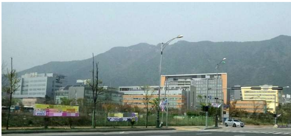
Figure V.4 Buildings of ‘D’ Hospital 193
