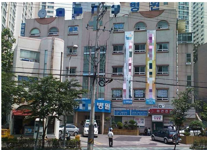
Figure V.3 The Front View of ‘C’ Hospital 185
