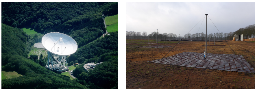
Figure 1.5: Left : Single dish radio telescope in Effelsberg, Germany [Credit: Dr. G. Schmitz, downloaded from de.wikipedia.org/wiki/Radioteleskop_Effelsberg ]. Right : LBA Antennas of the LOFAR station “DE609” in Norderstedt, Germany [Downloaded from www.glowconsortium.de ].
