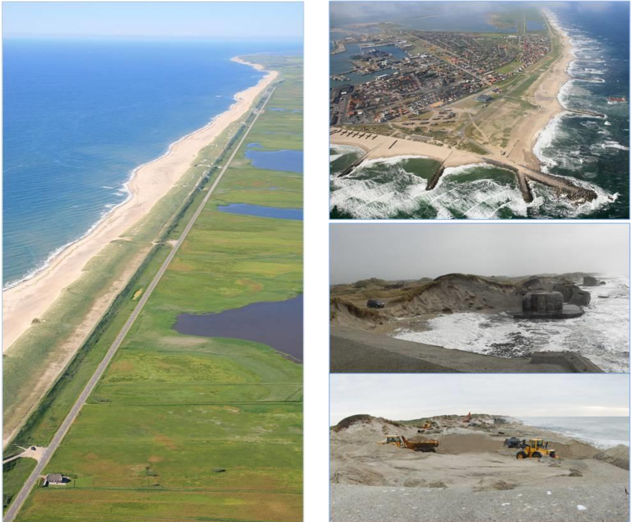
Fig. 8: Dike and artificial dunes north of Thorsminde (left), groins and sea dike at Thyborøn (top right), and storm erosion and dune repair north of Hvide Sande
