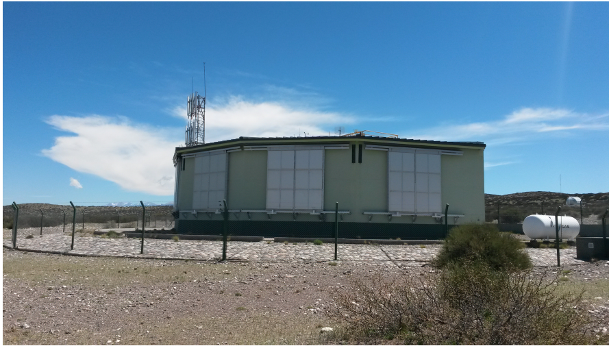
Figure 5.2: A photography of the FD building Coihueco taken during daytime, hence the closed shutters in front of each bay. The white building in the background to the right of the FD building is the lidar station at the site of Coihueco.
