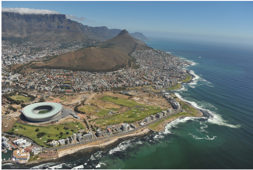
Figure 25 Aerial photograph of the Cape Town Stadium
