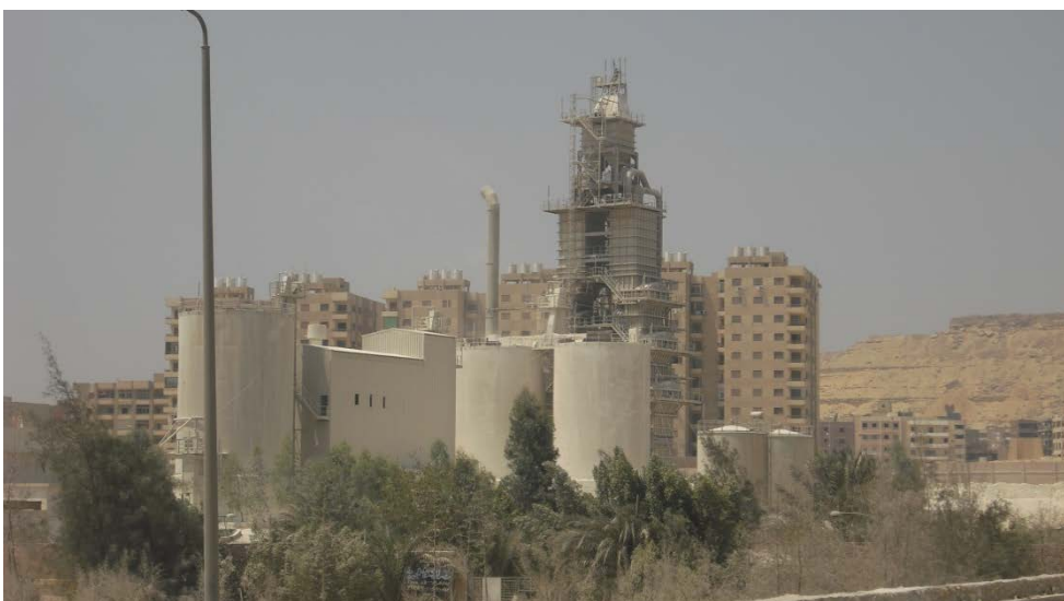
Figure 89: Cement factory along autostrad road close to recently settled areas. Photo captured 2010
