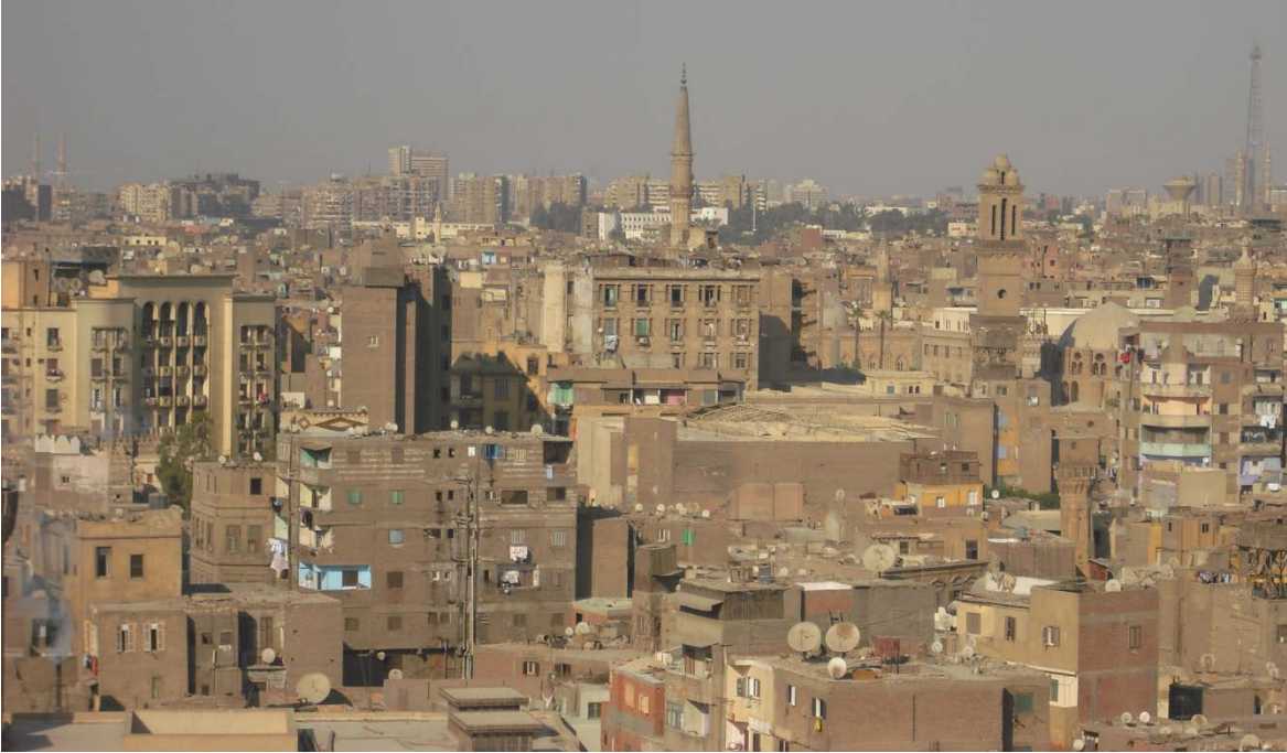
Figure 119: High density urban area in GCM core showing heritage buildings. Photo captured 2010
