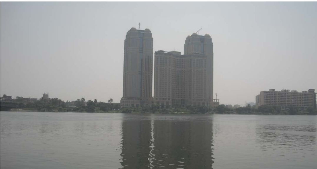
Figure 120: New towers on the Nile River show the replacement process and the transformation of urban patterns. Photo captured 2010
