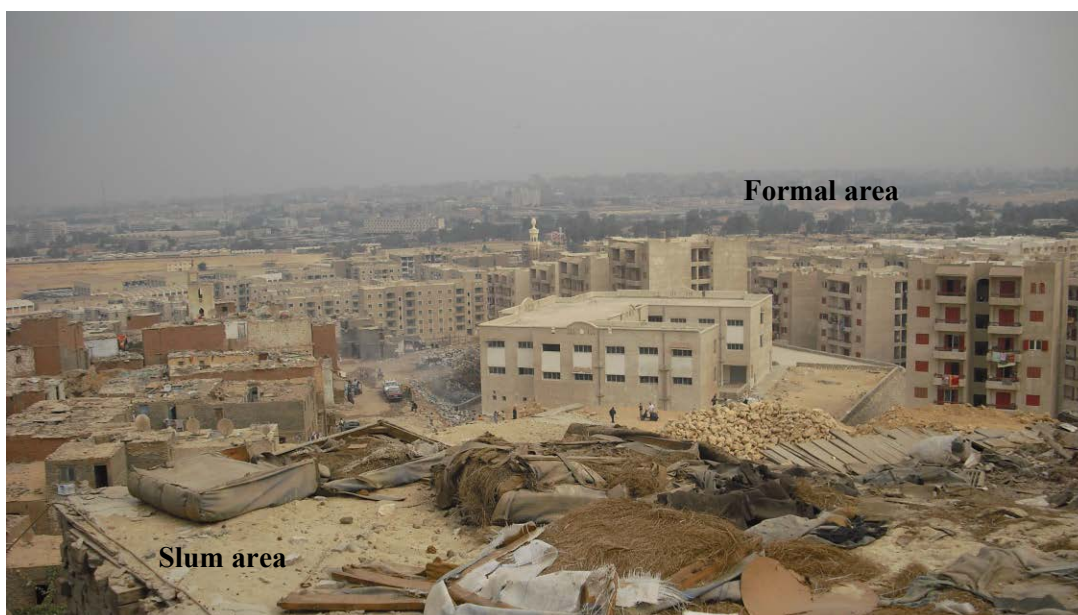
Figure 124: The limitation of slum expansion due to the formal project. Photo captured 2010
