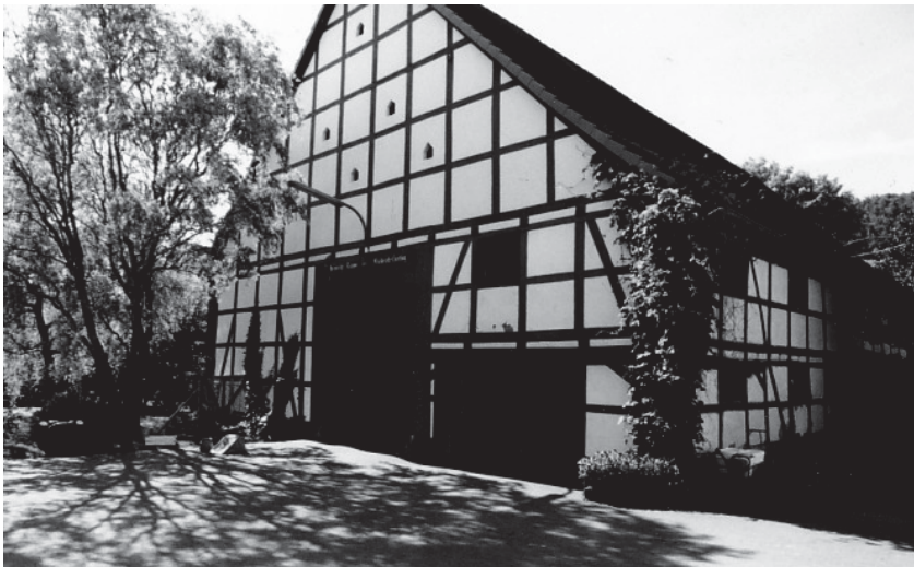
Warbsen, Forstbachtal 9, Scheune, S-Giebel
