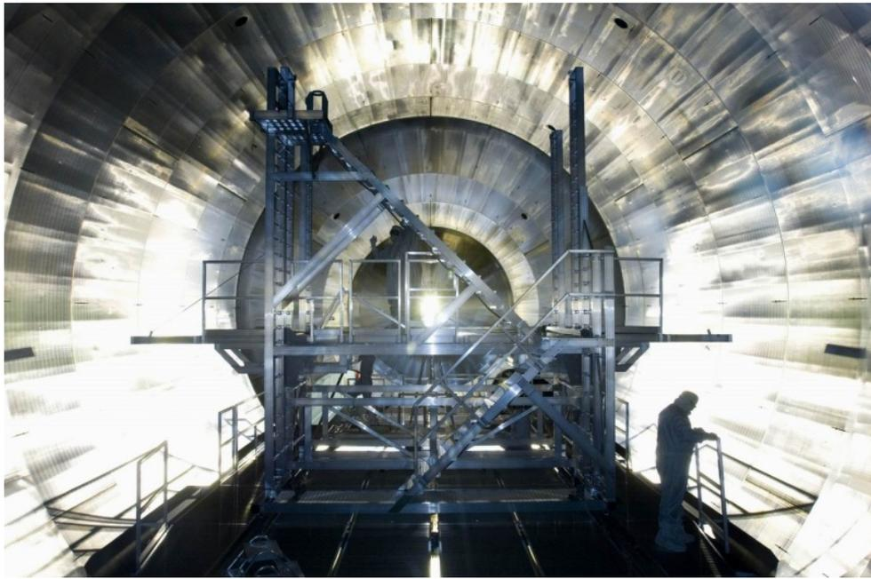
**Figure 4.28:** Scaffolding and working platform for the installation of the inner electrode system inside the main spectrometer vessel (June 2008). Photograph: FZK.
